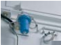
Leakage detector and cooling air temperature detector
